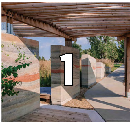
RAMMED EARTH WALL COMBINES BUILT STRUCTURE WITH NATIVE ENVIRONMENT SHOWCASING NATURAL PATTERNS EL MURO DE TIERRA APISADA COMBINA LA ESTRUCTURA
